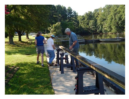
Each old decking board is used as a template for its replacement board for cutting to length and pre-drilling holes for fasteners.
